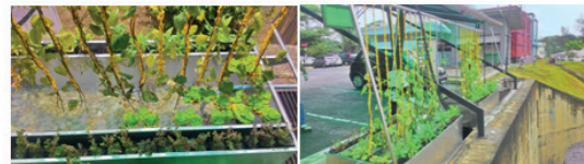
Figure 2: VGS Installation on the Car Park Structure
